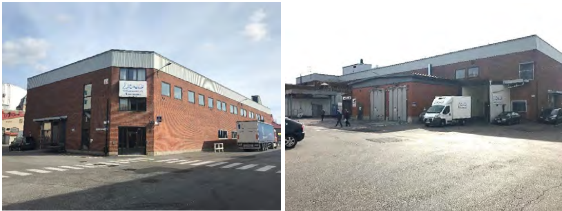
Figure 1 Exterior of the building in Hallvägen 7 A-C, Hallgränd 2-4
